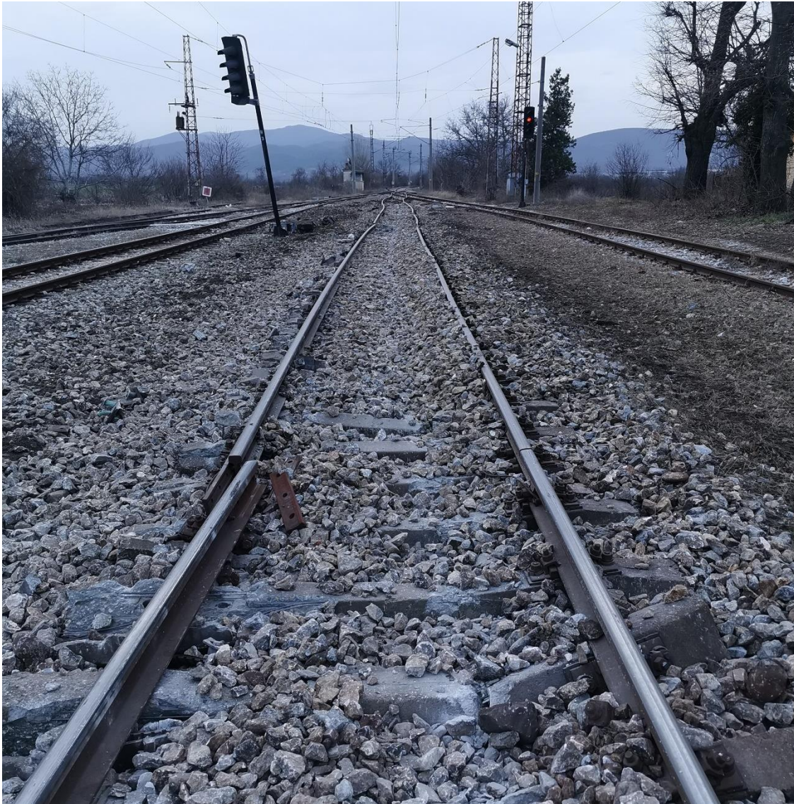
Fig. 4.21. View from second track to switches №№ 2 and 4.
