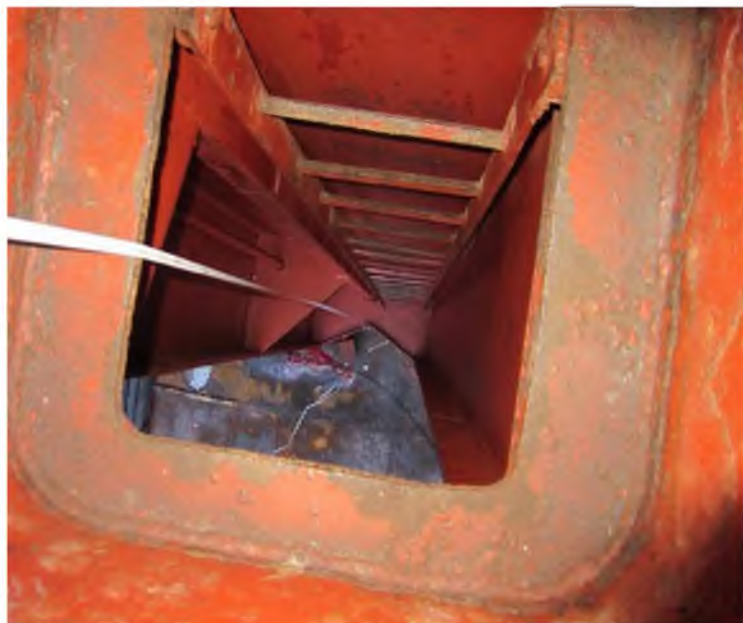
Fig. 3 Entry to the vertical ladder, upper part.
