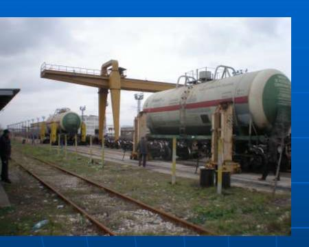
Track for replacing the undercarriage of railway cars with hazardous cargo — with standard-gauge tracks, and two stations fitted with explosion-proof jacks. The yard can handle up to 20 railway cars in 24 hours.
