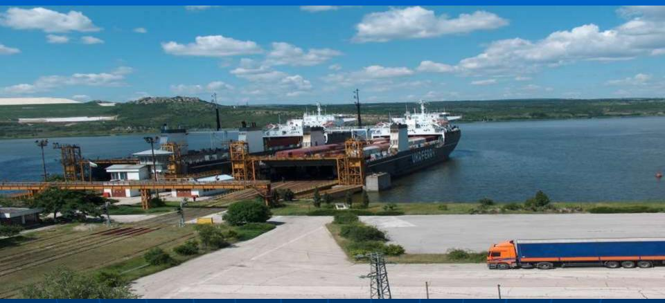
The Ferryboat Terminal Varna has two berths, equipped with bridge gantries with five 1520 mm railway tracks each. The ferryboat terminal has the capacity to handle a ferryboat carrying 108 railway cars for 10 hours, and a ferryboat carrying 45 railway cars for 2 hours. The berths can accommodate two ferryboat vessels, 26 m and 22 m wide, respectively.
